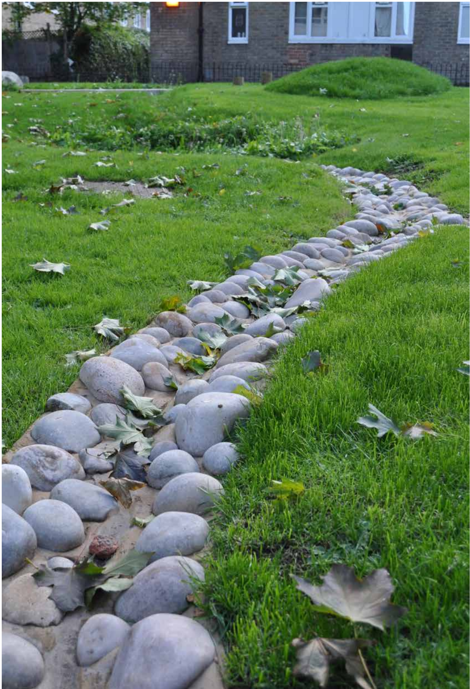
Paved & planted drainage channels
