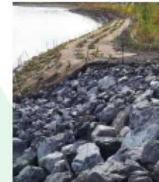
Planting saltmarsh in geotextile membrane © City of Calgary, 2019
