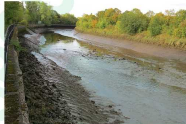
Canalised banks of the lower River Derwent - looking south
