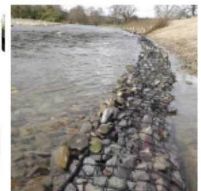
Rock rolls to create terraced steps to trap sediment and develop saltmarsh
