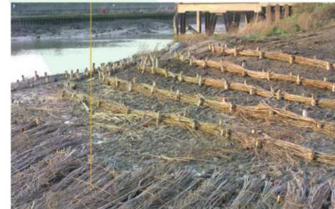
Brushwood mattress comprising fascines / faggots held by a grid of fixing posts
