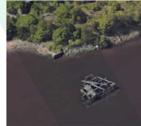
Derelict timber dolphin structure could support a tern nesting island
