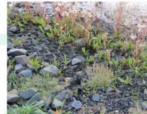
Saltmarsh growing in plastic geotextile membrane
