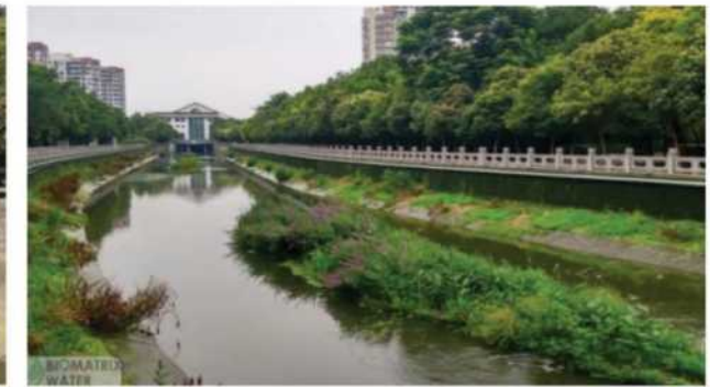
Examples of canalised river restoration with floating riverbanks and island modules © Biomatrix
