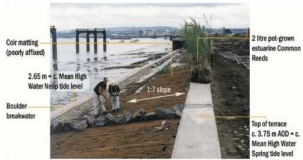
Eastern wall, Greenwich Peninsula, London: Site 2 during construction
