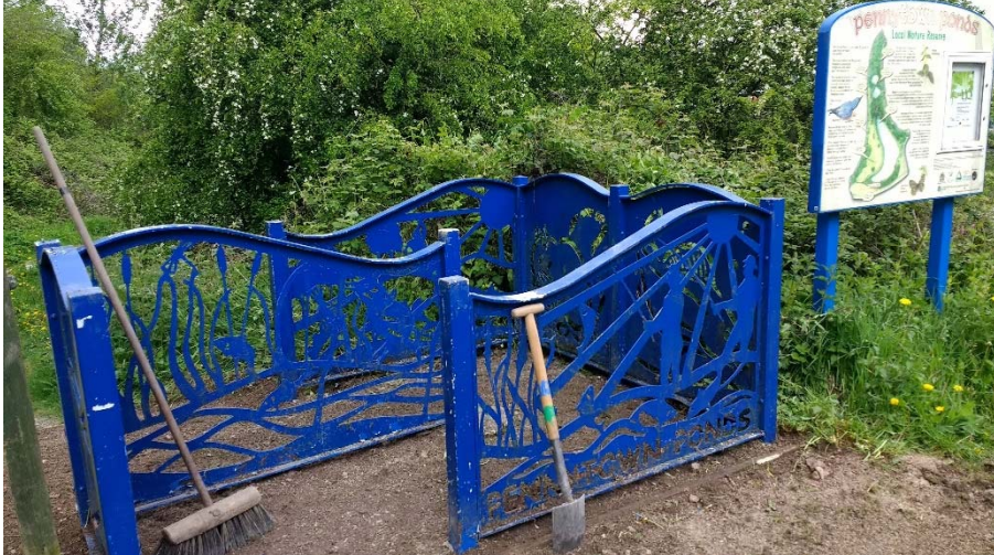
Clearing vegetation around main entrance gate
