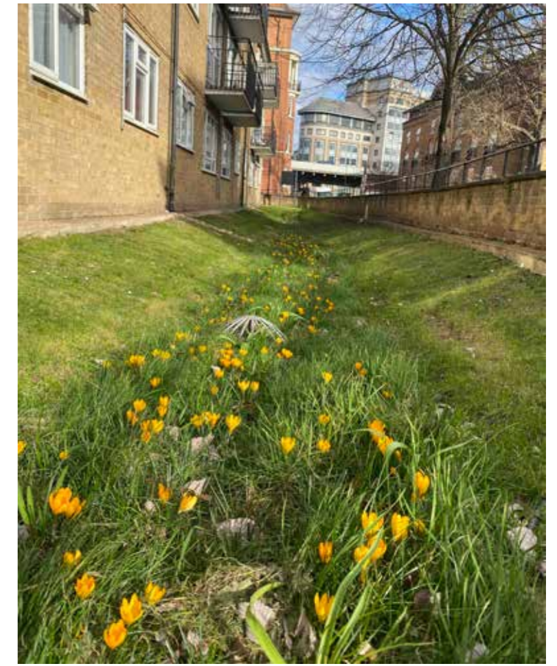
2.5m wide / 300mm deep bioswales could move water around the site, provide a boundary feature and a new plant community, such as wildflower or bulb planting.
