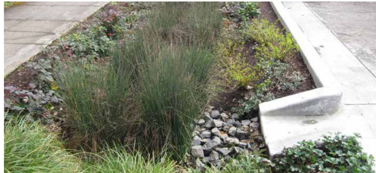
Reduce on-street parking by introducing kerb side rain gardens that collect rain water and bring it into the greenspace.
