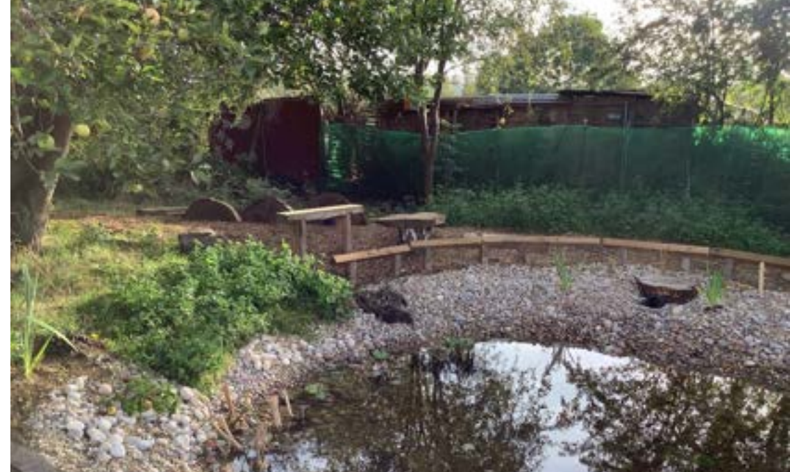
The original leaky pond was replaced with two new ponds
