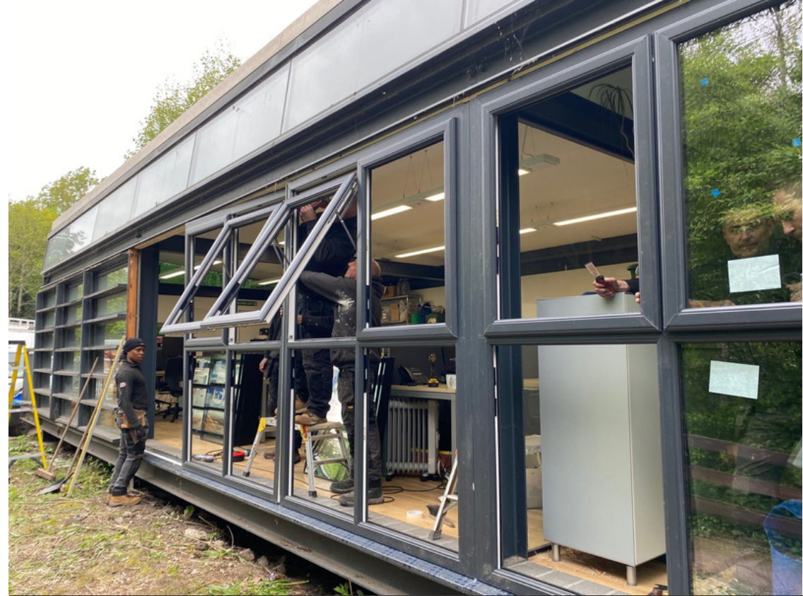
Double glazing being installed at Ecology Park office
