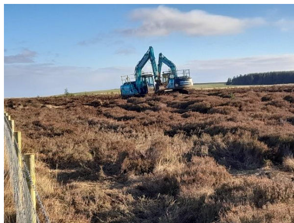
Stump-flipping and infilling drains to restore bog conditions
