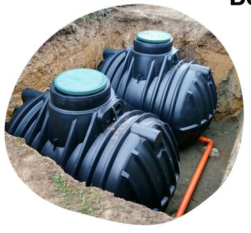
The school has a built-in system to harvest rainwater. This collects water from the roof and stores it in an underground tank. The water is then pumped into the school where it is used to flush toilets and urinals, and to water the garden.
