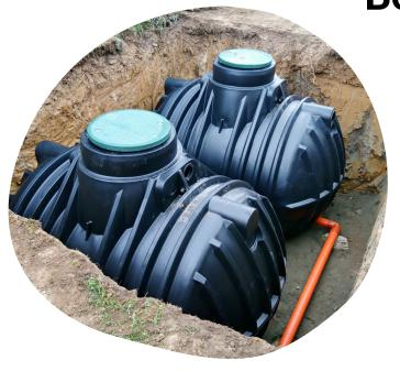
The school has a built-in system to harvest rainwater. This collects water from the roof and stores it in an underground tank. The water is then pumped into the school where it is used to flush toilets and urinals, and to water the garden.
