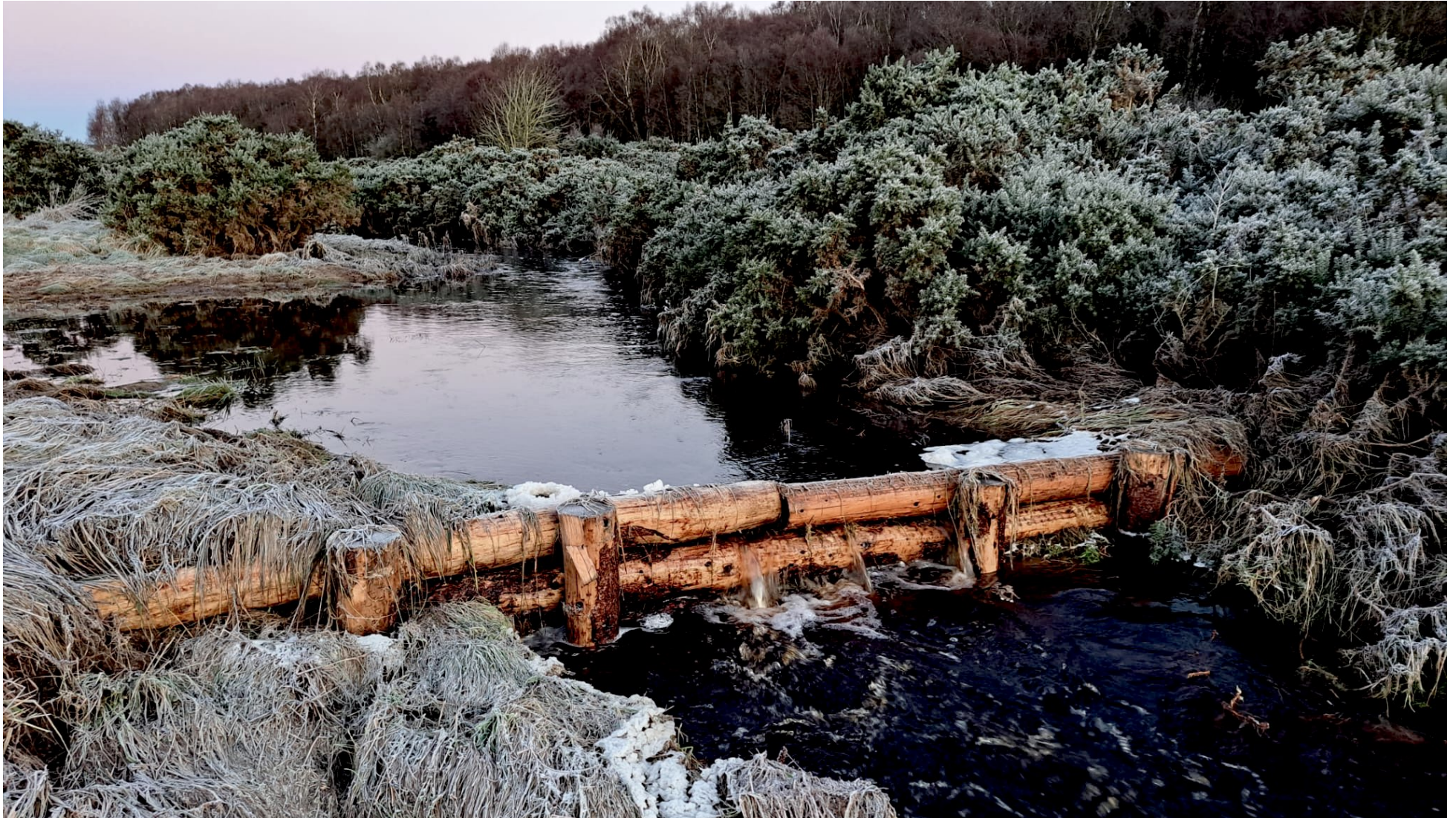
➤ LEAKY DAM INSTALLED AT HARWOOD BURN (GALLOWES HILL)
