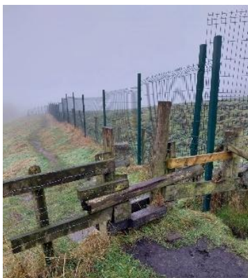
Fig 6a: Damaged stile
